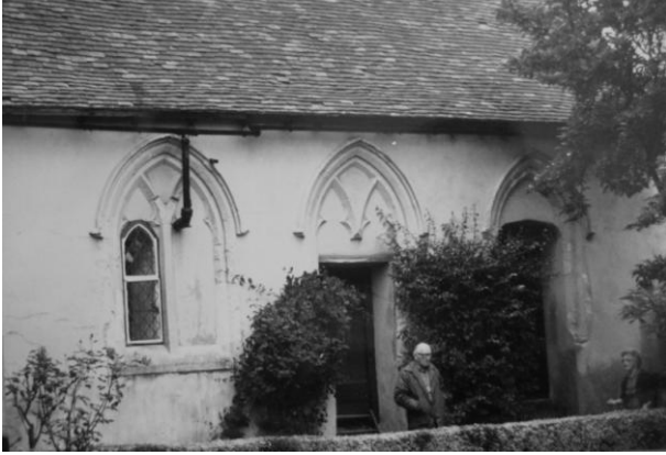
The exterior of the chapel
